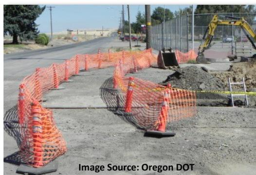
Obsolete "Work Area Fencing" shall **not** be used as channelizing devices. This fencing does not provide pedestrians with adequate protection from work area activities or traveling vehicles and does not provide a continuous, detectable bottom edge.
