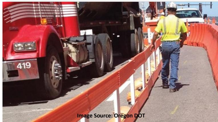
Above, the pedestrian route is delineated on both sides to provide a physical barrier between the pedestrian and the work zone as well as between the pedestrian and vehicle traffic.
