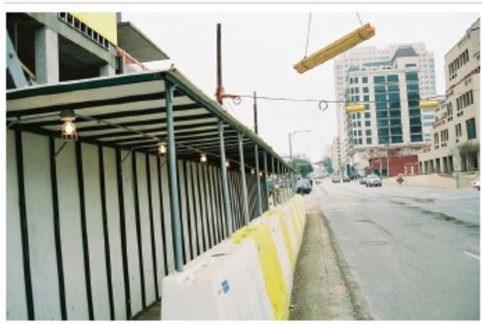
A covered walkway protects pedestrians from construction dangers occurring above them including falling debris. Covered walkways shall be lit for nighttime use and include proper barriers along their alignment.
