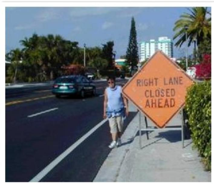
The above sign places the pedestrian in immediate danger by forcing the pedestrian onto the roadway to navigate around the work zone warning signs. This type of sign placement shall not be used.
