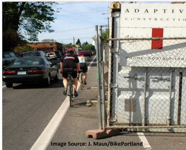
No channelizing devices are provided for cyclists, forcing them to squeeze between the work area and the travel lane for motor vehicles. No signage or bicycle specific accommodations are made.
