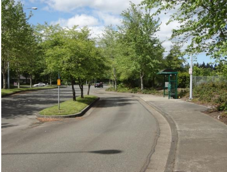
Bus Pullout with Longitudinal Island
