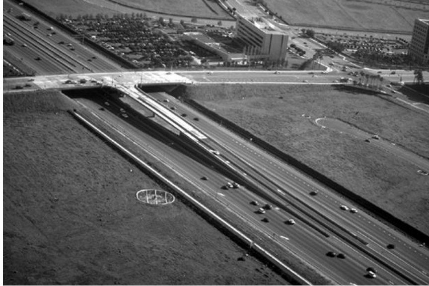
Drop ramp photograph from FHWA/PB HOV Interactive 1.0 High Occupancy Vehicle Data Base from the U.S., Canada, and Europe
